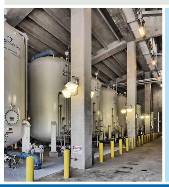
three nozzles along the straight side of the vessel can be fitted with in-bed sample assemblies to allow the operator to monitor the progress of the adsorbate as it flows through the bed.
